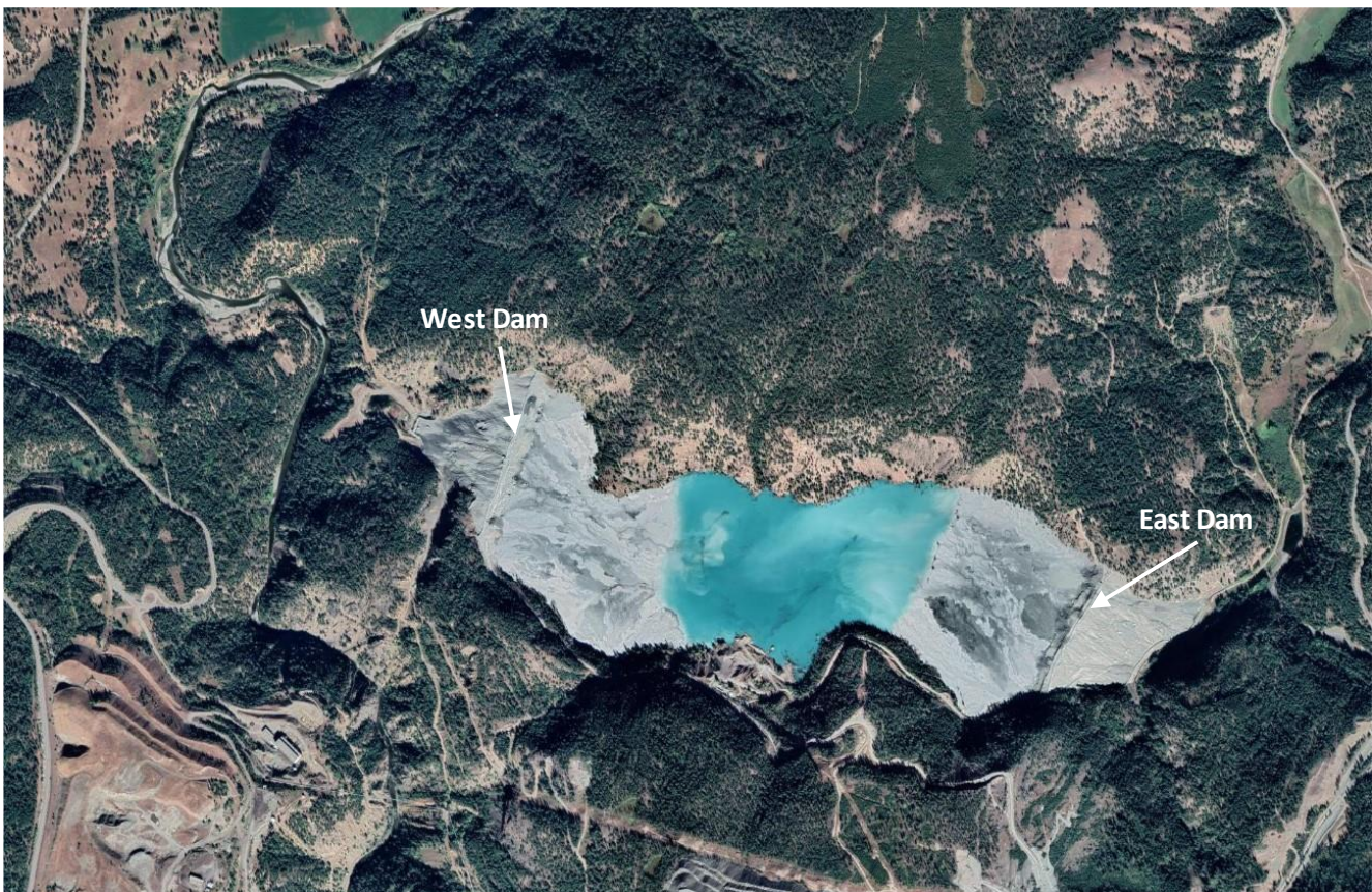
Figure 1-1. Aerial view of the Copper Mountain Mine tailings storage facility, with west and east dams above the Similkameen and Wolfe Creek drainages, respectively.
